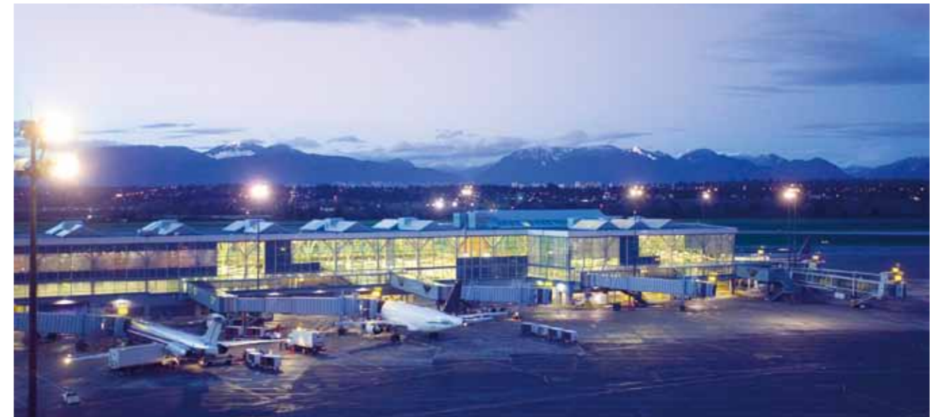
▲ Airports have multiple stakeholders, who require different authorization levels and customized GUIs for PSIM access.
